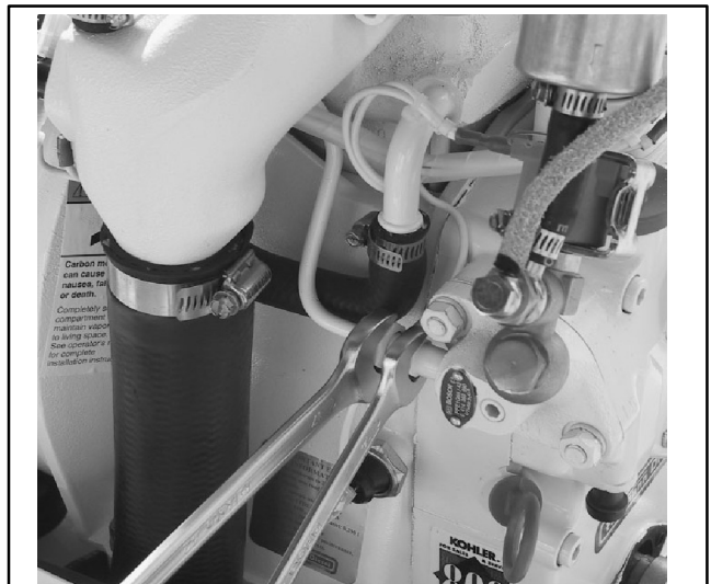
Figure 10-28 High-Pressure Fuel Line on the Delivery Valve
